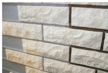
The installed clinker façade tiles along with grouting joints on the insulating panel
